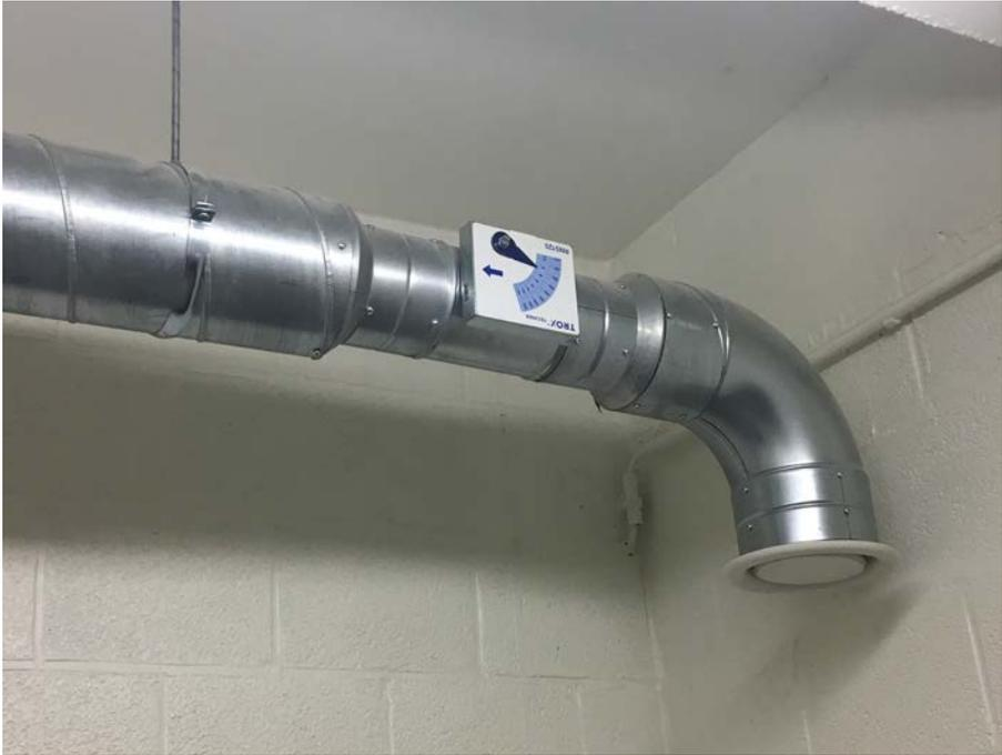
*FIG. 19. Piping of the ventilation system to maintain negative pressure in order to reduce contamination and internal exposure of workers when working with aerosols or volatile radionuclides. (Courtesy of the Department of Medical Imaging and Small Animal Orthopaedics, Faculty of Veterinary Medicine, Ghent University.)*
