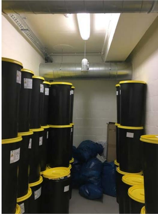
*FIG. 20. A storage room for radioactive waste. Contaminated waste needs to be stored separately, preferably in a separate room. Walls and floors need to be washable and non-porous. The transitions between wall and floor need to be seamless. Note the piping of the ventilation system at the ceiling to maintain negative pressure and to prevent internal contamination of workers.*
