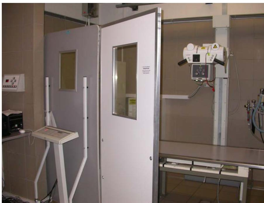
*FIG. 4. Use of a protective barrier (shielding screens) placed at the control console to reduce exposure of the operator when performing X ray examinations. (Courtesy of the Department of Medical Imaging and Small Animal Orthopaedics, Faculty of Veterinary Medicine, University of Ghent.)*
